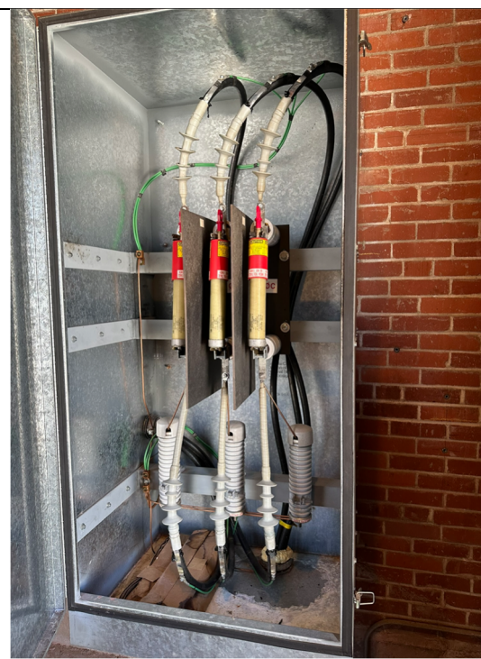
Mech Room 4-04: Primary fusing
